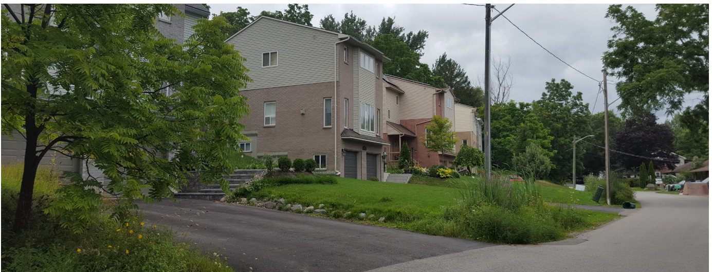
Looking at the most recent development on Old Main Street between #198 and 210B Old Main St
