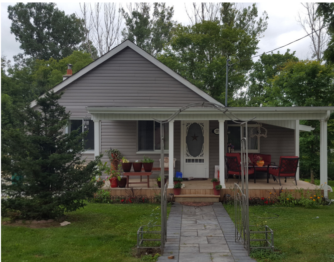
Example of an intermediate roof pitch above the entrance
