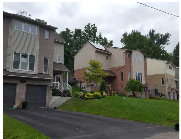
Disconnected ground floor condition
