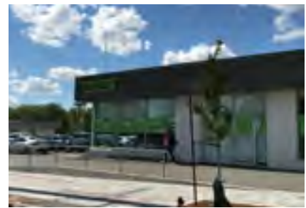
Commercial / Office on Davis Dr
