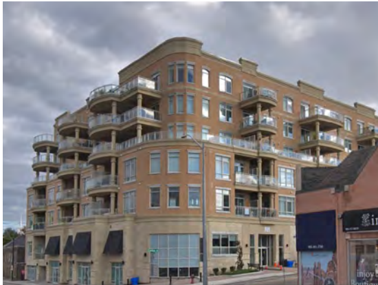
15277 YONGE STREET, AURORA Five Storey Mixed-Use Building Population 1 : 160 Jobs 2 : 60 Gross Area 3 : 0.5 ha
