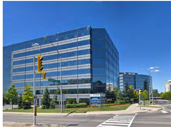
55-198 COMMERCE VALLEY DRIVE, MARKHAM Eight, Nine Storey Office Buildings Population 1 : n/a Jobs 2 : 4,900 Gross Area 3 : 13.8 ha
