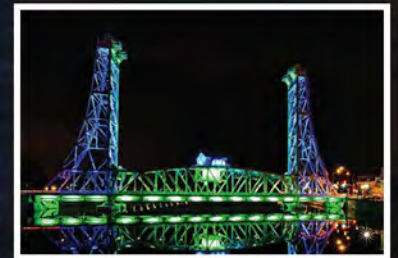
Welland Bridge 13 Photo courtesy: Anthony Gallaccio
