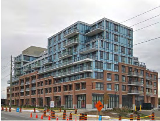
11611 YONGE STREET, RICHMOND HILL Eight Storey Mixed-Use Building Population 1 : 415 Jobs 2 : 70 Gross Area 3 : 1.2 ha
