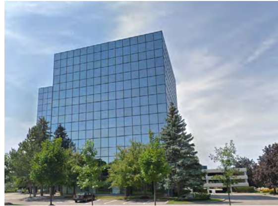
100 ALLSTATE PARKWAY, MARKHAM Eight Storey Office Building Population 1 : n/a Jobs 2 : 805 Gross Area 3 : 1.3 ha
