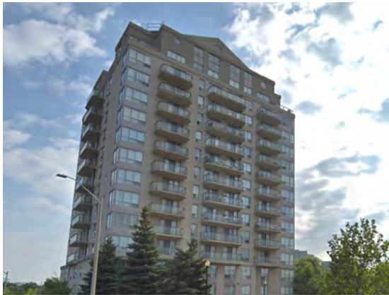
399 SOUTH PARK ROAD, MARKHAM 14 Storey Residential Building Population 1 : 215 Jobs 2 : 10 Gross Area 3 : 0.6 ha
