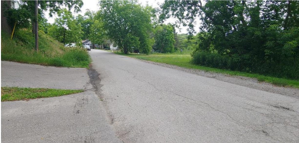
Image 9 Lawn beyond disturbed right-of-way, between forested road swale and sanitary sewer adjacent 205 Old Main Street North requires Stage 2 survey
